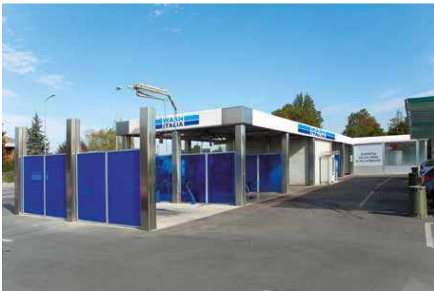
Pista esterna con parattia Uncovered bay with lateral protective wall
