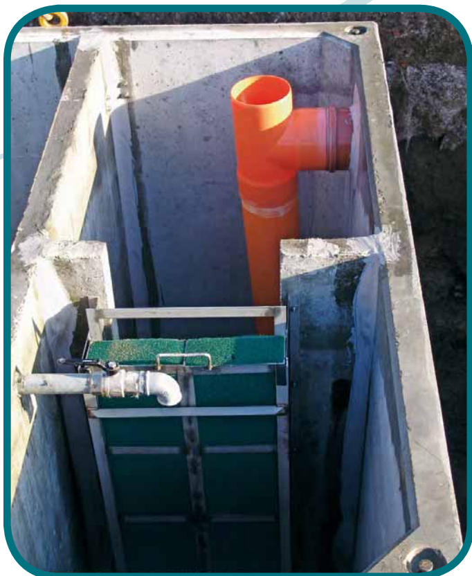
Dettaglio del filtro a coalescenza Detail of coalescence filter
