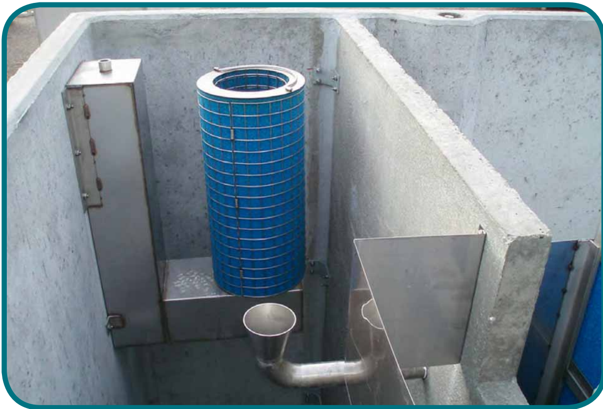
Particolare otturatore meccanico con relativo pannello a coalescenza View of the internal sections with the automatic oil interceptor and coalescence panel
